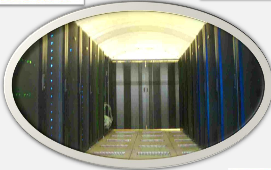
High Density Heat Containment System
