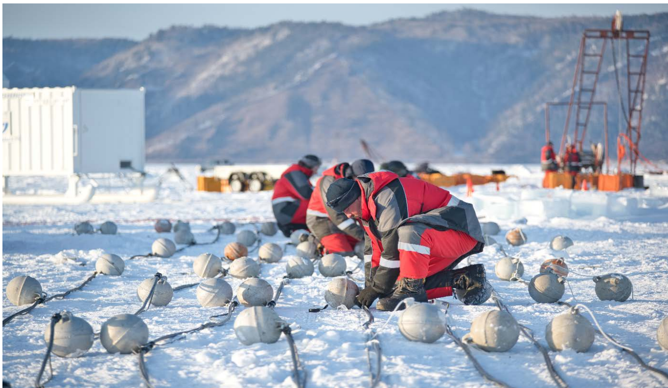
Fig. 12. Assembling the Baikal-GVD installation cluster garland
