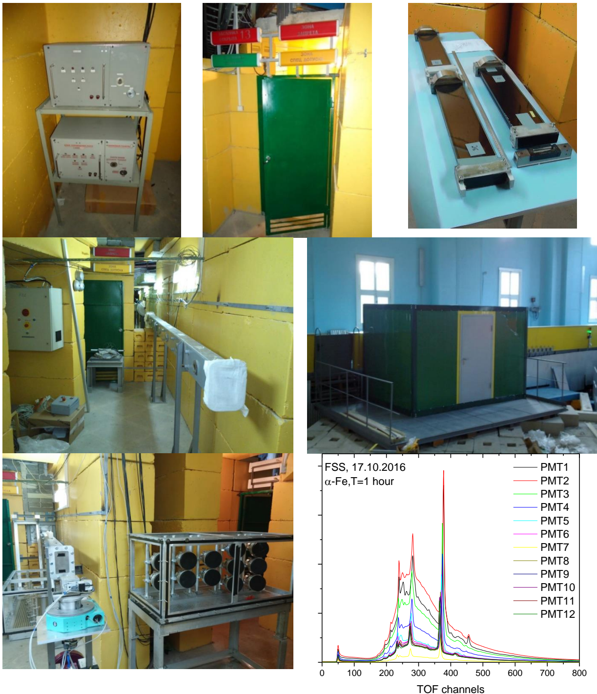
Fig. 45. Fourier-diffractometer FSS on IBR-2 beamline 13 (from top to bottom and from left to right): operational control boxes of a shutter and beam stopper; entrance door to the bunker (beam exit location); glass mirror neutron guide sections before installation in a housing; neutron guide installed in a steel housing and control electronics of the Fourier chopper; experimenter's control cabin mounted on the biological shielding of beamlines № 13-14; detector Ost (without shielding) after installation and alignment of 12 PMTs with glued ^6\text{Li} glasses; at the sample position, modules of the HUBER goniometer are installed and adapted to the FSS table; TOF spectra from standard \alpha -Fe sample measured by each of 12 PMTs of the 90^\circ -detector Ost at FSS.
